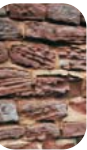
Local sandstones of variable quality have been used for the older cottages. At point 10 note the random stone on one wall and trimmed "rusticated" stone on another. A barn near the church shows serious weathering of the softer layers within the stones.
