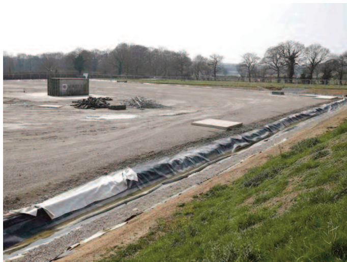
This is all there is to see currently at Horse Hill, a sea container over a capped wellhead.
